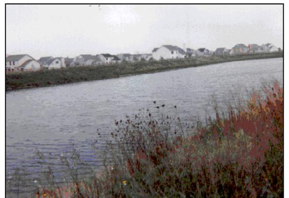
*Cell I of the odor-free, 650,000 gallons-per-day capacity deep-cell wastewater treatment facility at Mill Creek. Note the proximity of housing.*
