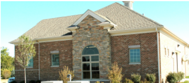
The Woods of South Barrington water operations building, viewed from the south.
